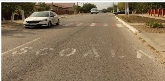
Picture 4. Road markings (Stage 1 countermeasures applied)
