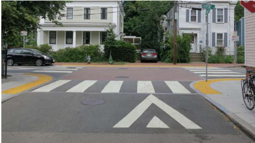
Figure 48: Example of raised pedestrian crossing. Source: Google photos
