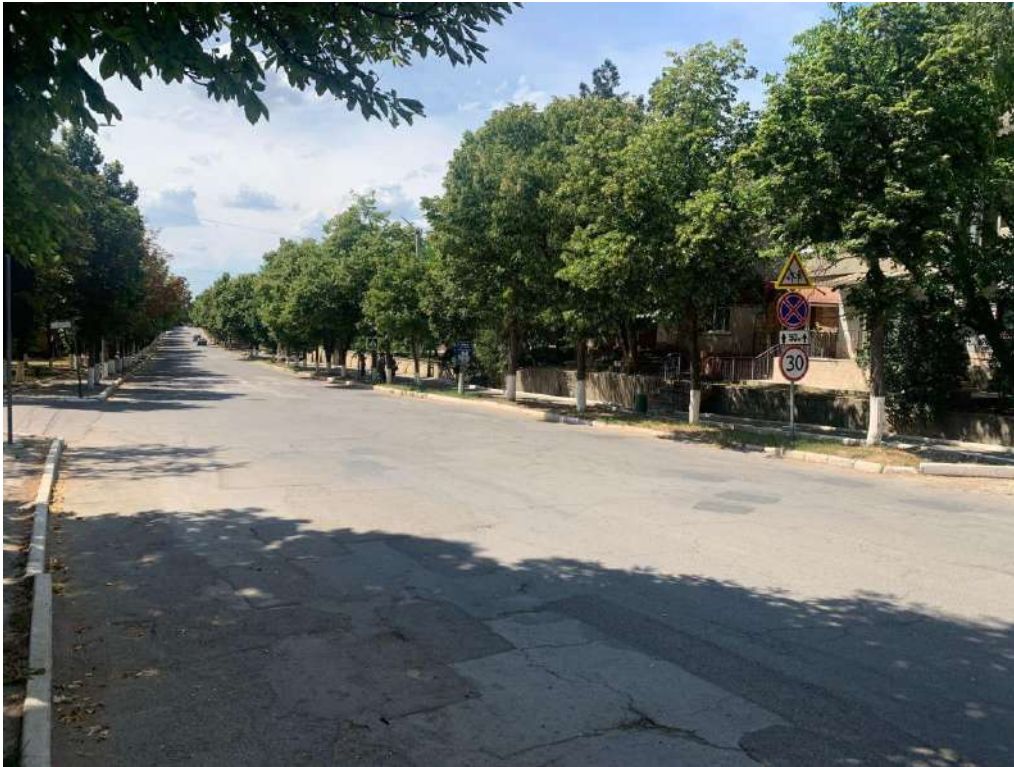
Figure 33: 30 km/h speed limit on Independentei street in Singerei
