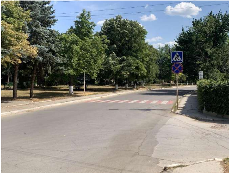
Figure 28: Pedestrian crossing in "Dimitrie Cantemir" school zone, Singerei
