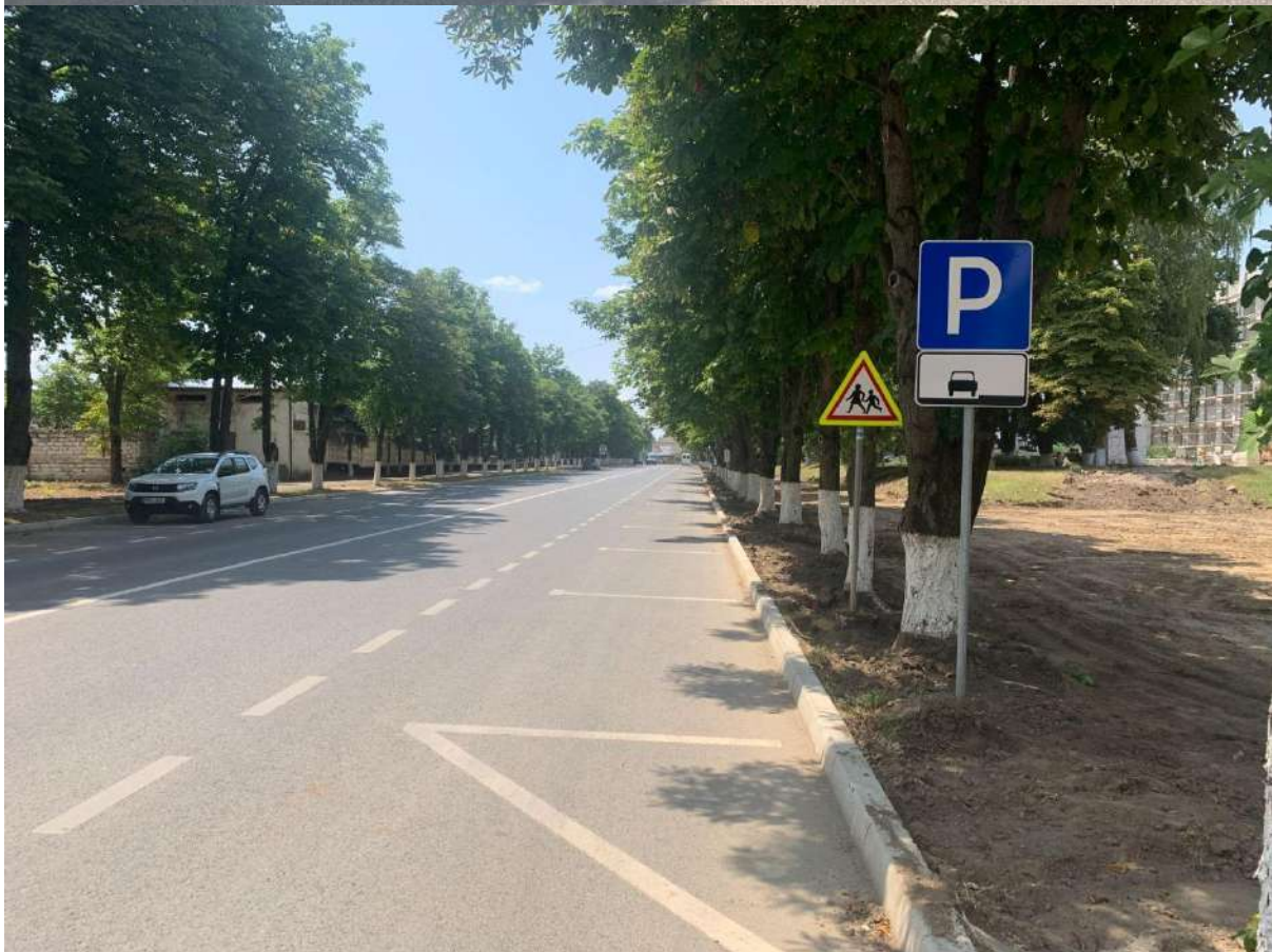
Figure 52: Parking mode, Nationala Street, Ungheni. Source: ACM
